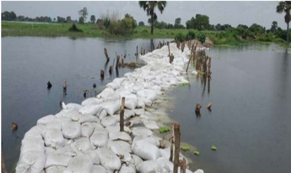
Figure 3: A dyke constructed in Makuach Payam, Bor County
